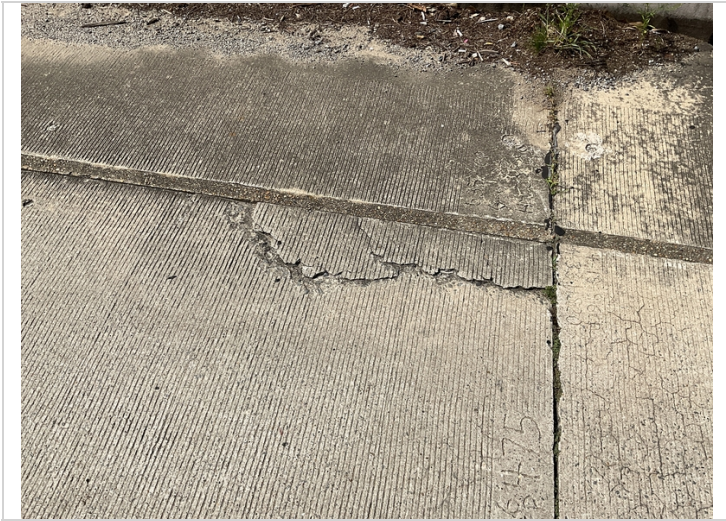
Span 3, channel unit 7 delam
