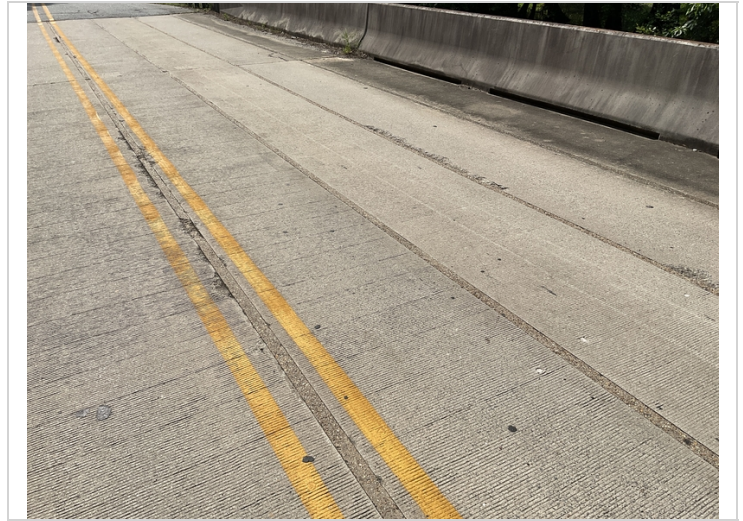
Span 2 units 3,4,5,&7 small spalls in units at grouted key ways.
