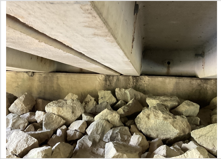
Bent 1 spalls under units 6&7
