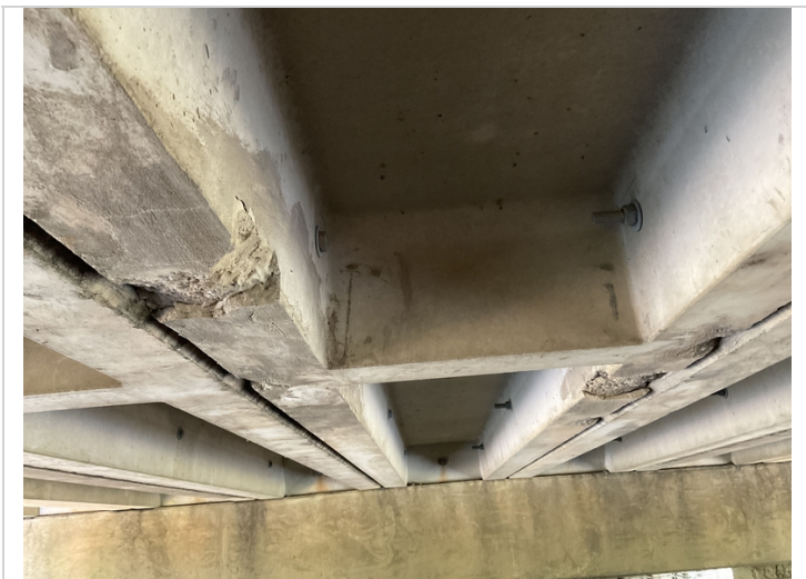
Span 2 unit 5 spalls on channel legs.
